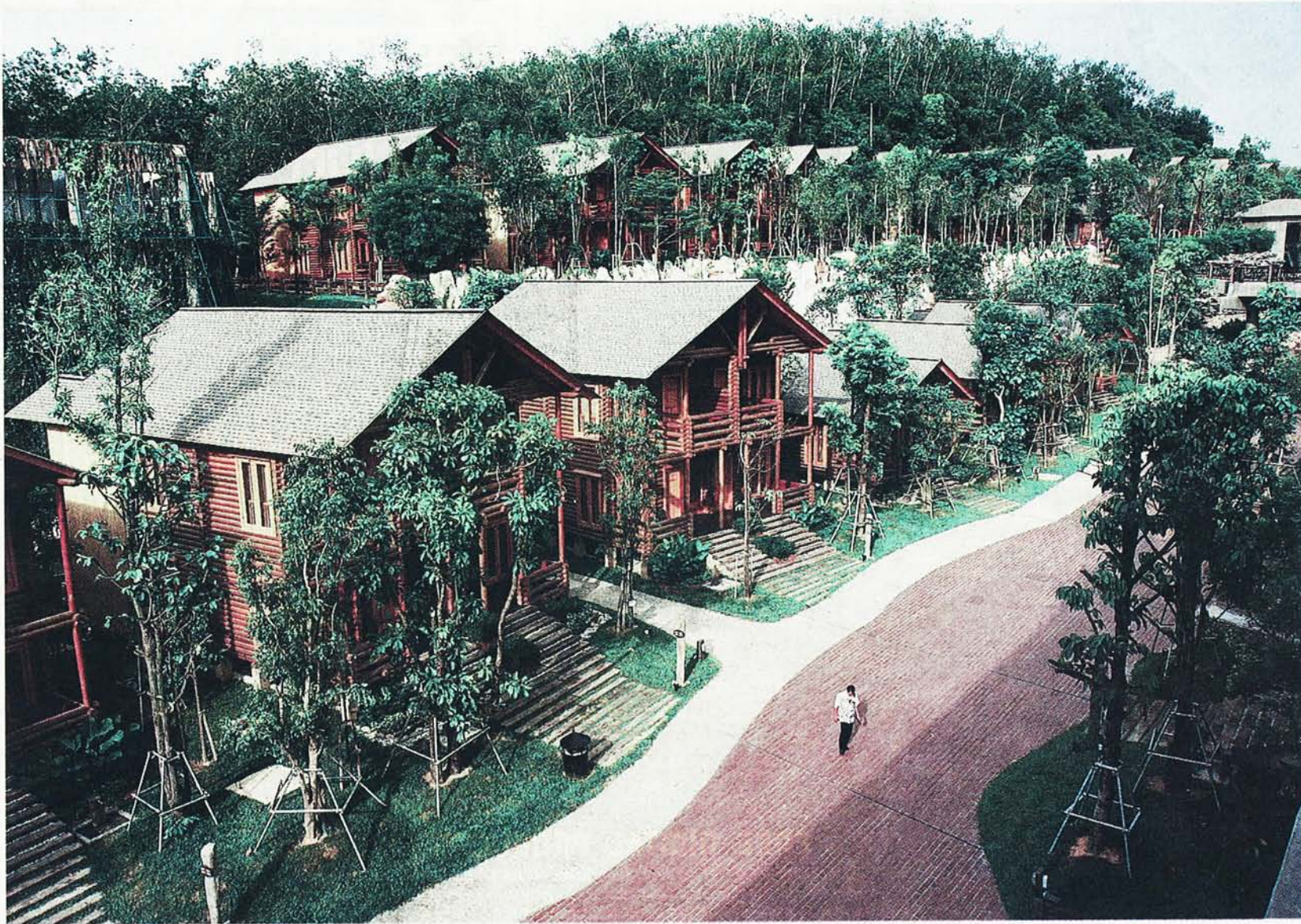
The units are built of pine imported from Russia. — Picture by Nashairi Mohd Nawi
